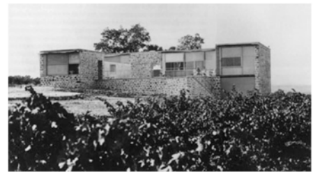
Fig. 5: "Primitive building techniques and sophisticated components appeared as expressive elements in Le Corbusier's architecture from the Maison Loucher onwards. We encounter comparable mixtures of off-site, in-situ construction in the shop-built timber windows and rubble-stone walling of the vacation house that he build for Madame Helene de Mandrot near Toulon in 1931" 21
